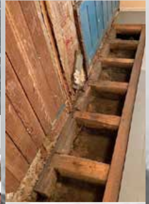
Floor joists in old original bedroom. All logs are hand hewn, notched, and set with no nails.
